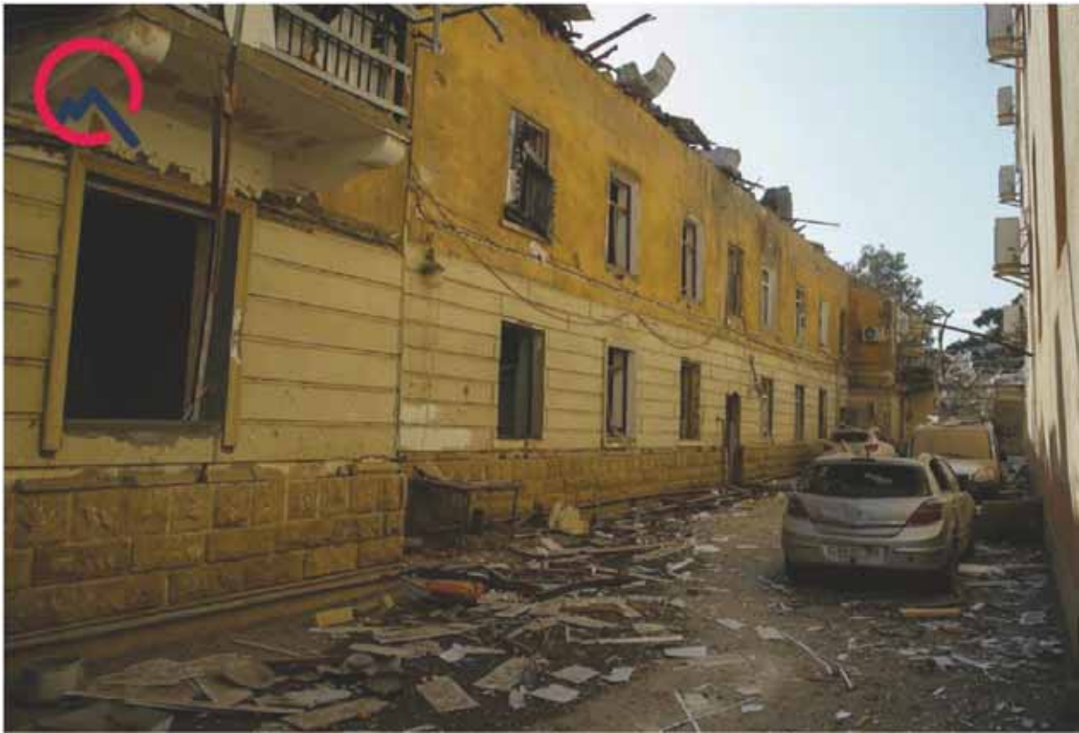
Damage inflicted upon the civilian infrastructure in the city of Ganja
