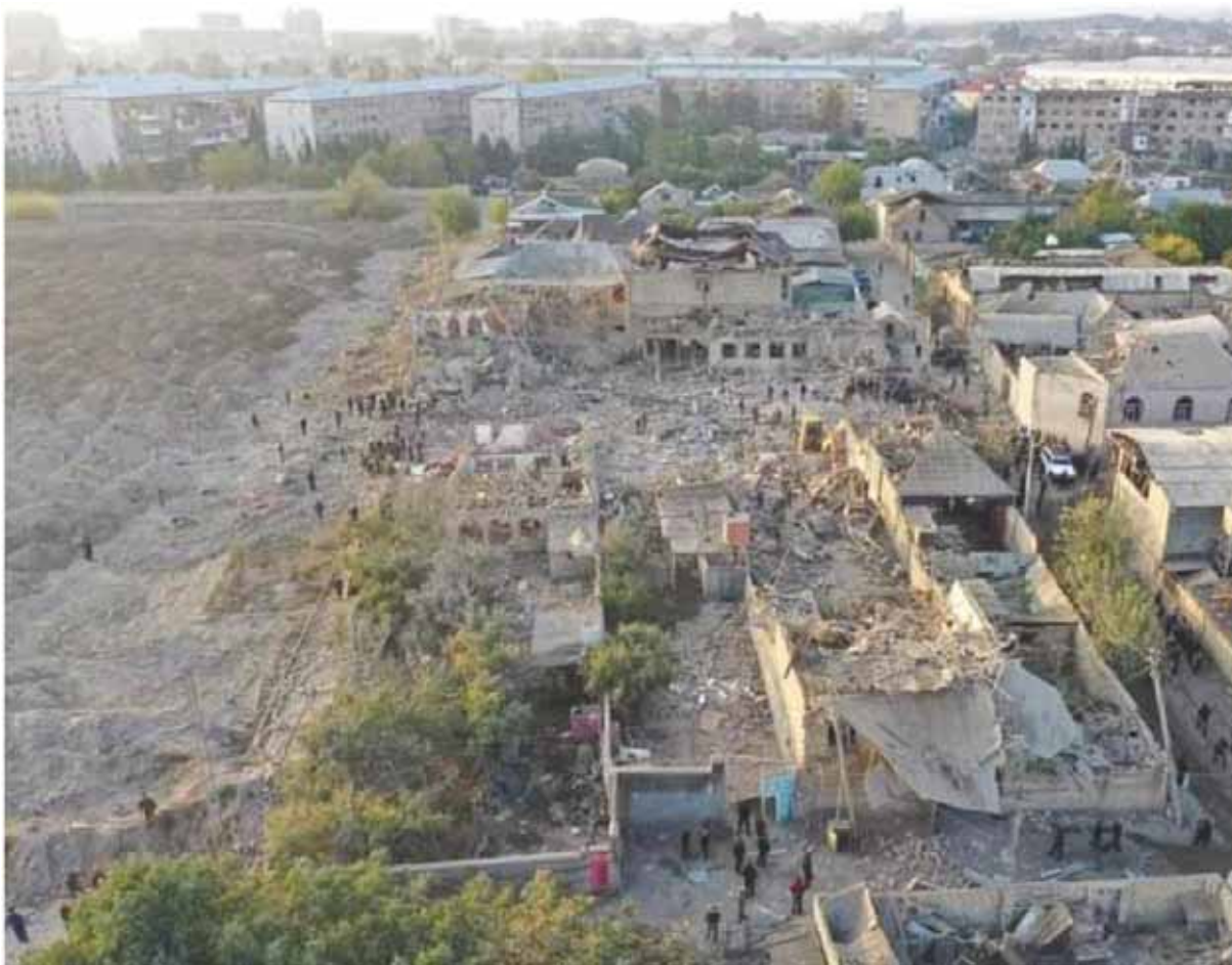
Destroyed residential area in Ganja (birdeye view)
