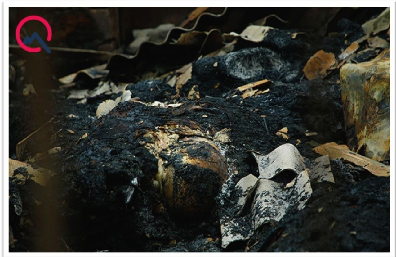
Photo 7 – 8: Private property damaged in the Aghdam district
