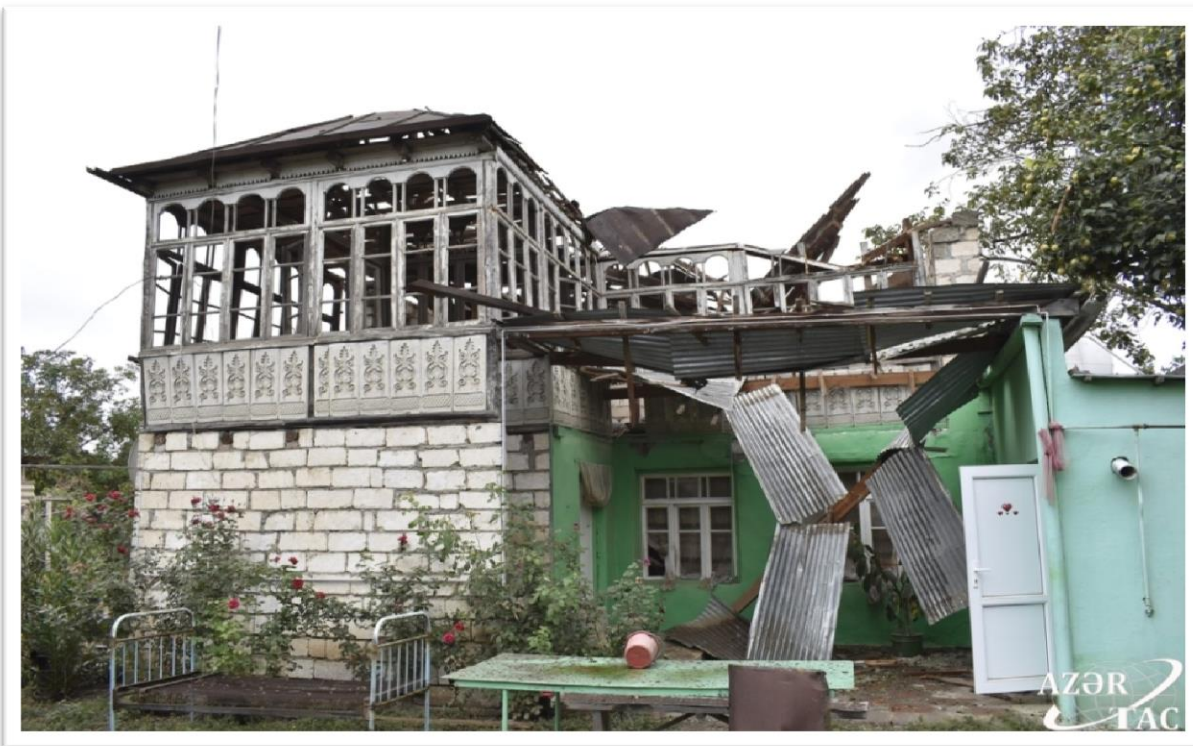
Photo 11 – 12: Private houses in the Aghdam district damaged
