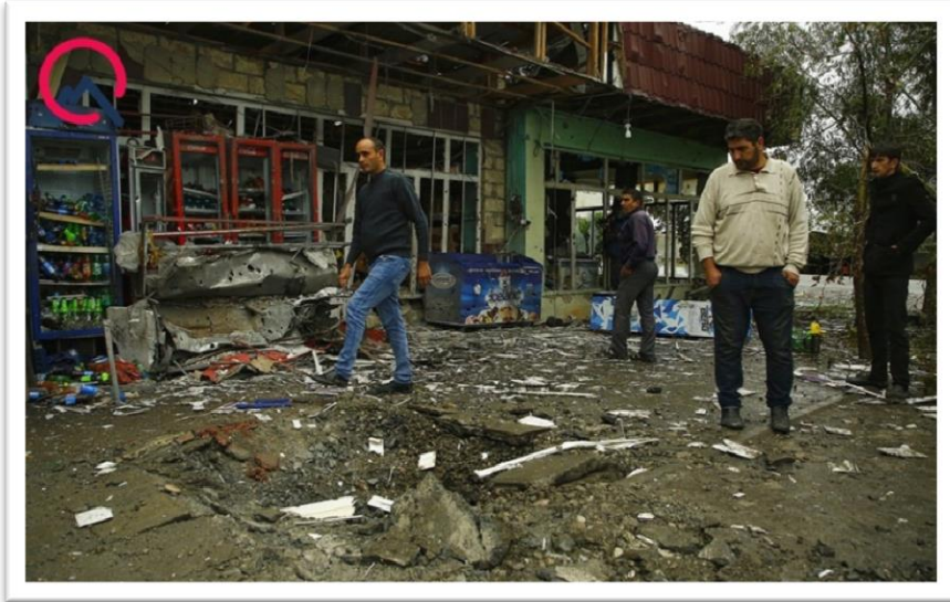
Photo 32: Local bazar consisted of numerous shops and markets were destroyed by artillery shelling
